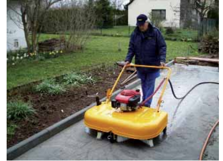
... brushing material in to the joints of the paving: the powerful Easy-Fill EF-H.
